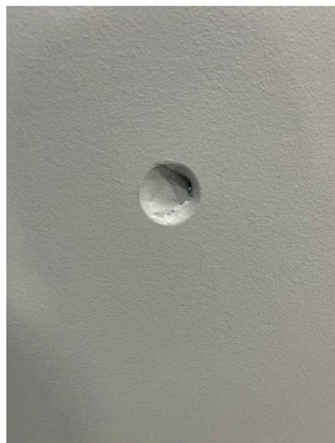
Wall had damage from doorknob. Possibly due to lack of door stopper. Recommend a qualified handyman or drywall contractor repair.
